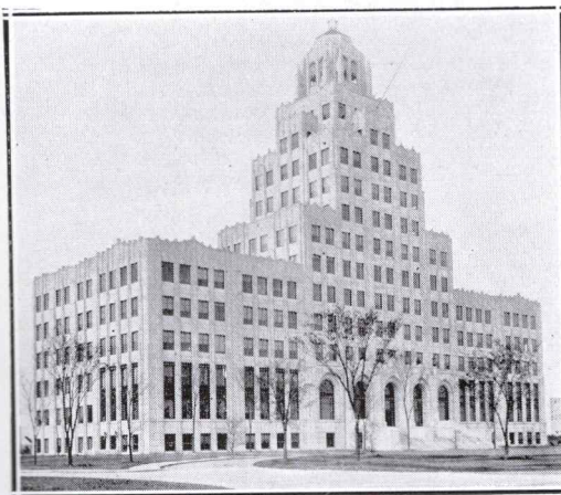
Staley Administration Building
